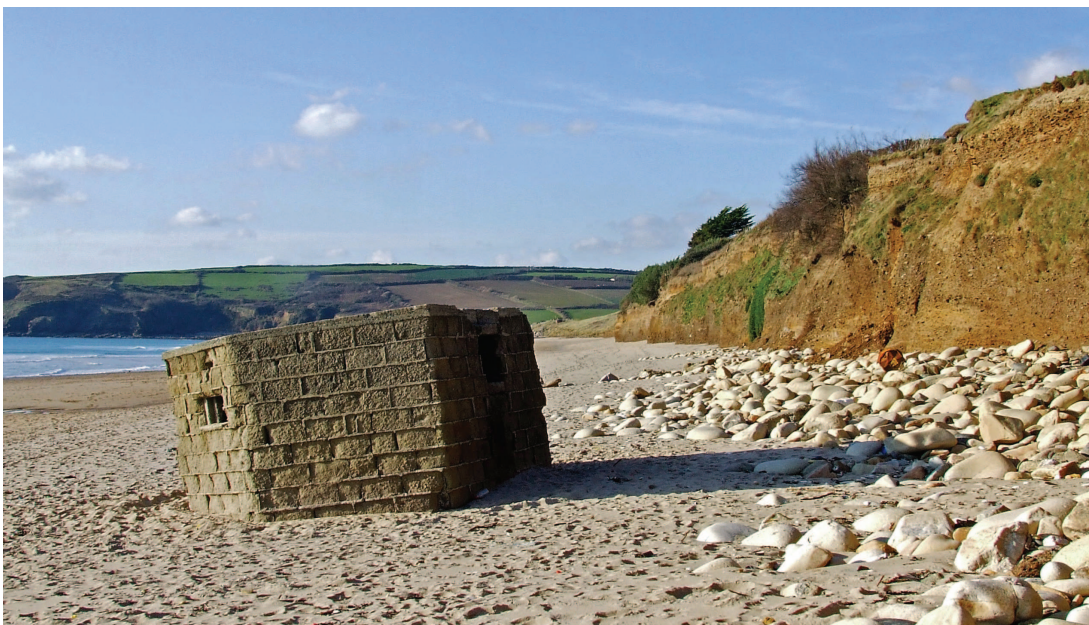
Erosion of the cliff by several meters has resulted in this World War II pillbox falling onto the beach. Such erosion could become more widespread with rising sea levels.
